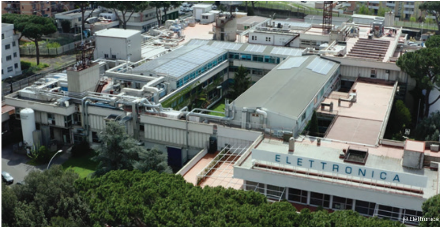
An aerial view of Eletttronica installations.
